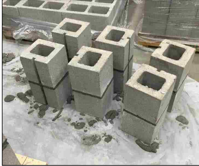
Figure 11. Masonry Prisms Prior to Grouting
