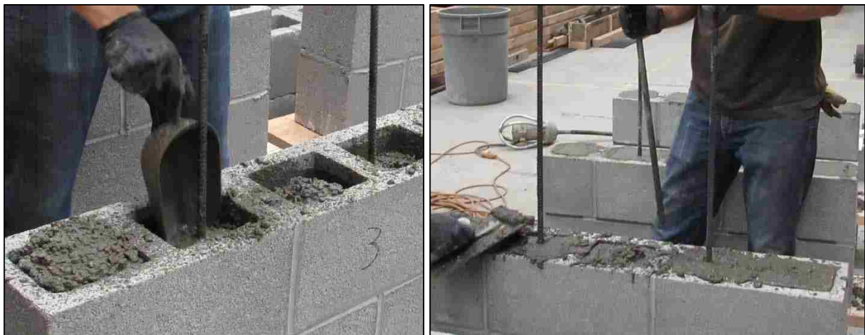
Figure 18. Filling Top Portion of Walette
