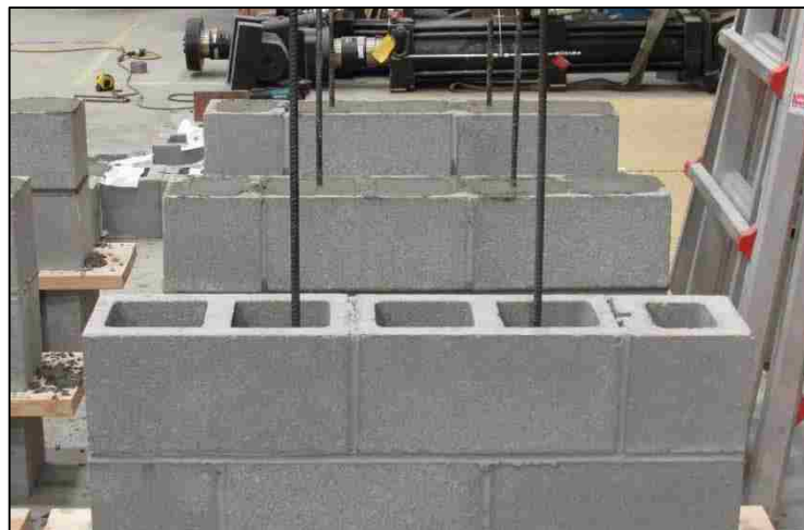
Figure 16. Placement of Reinforcement Prior to Grouting
