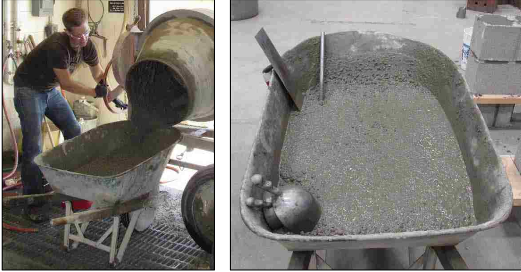
Figure 15. Grout Mixing and Composition
