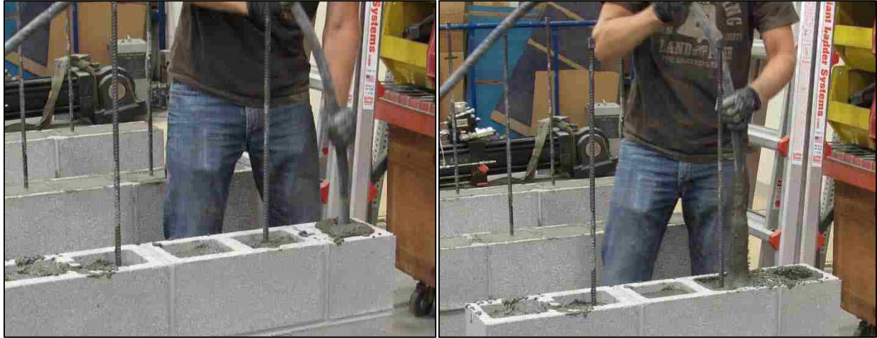
Figure 19. Consolidation of Grout using Vibratory Stinger
